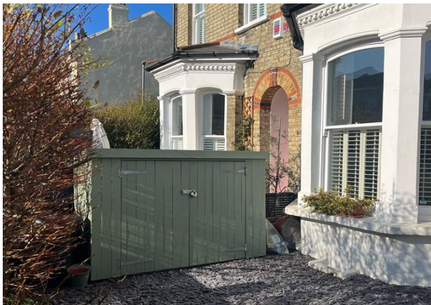
Figure 4 - External Bike Store (Metal) (Front)
